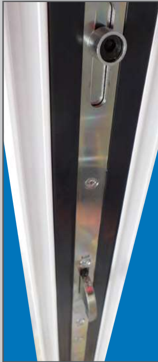
View of lower hook bolt and cam
